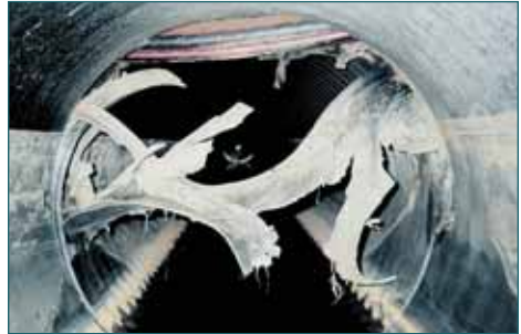
Trenched Power Cable.
