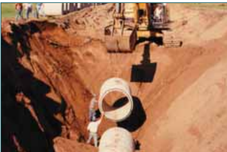
Concrete Pipe Installation.
