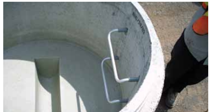
Figure 4 - Factory Produced Benchng
