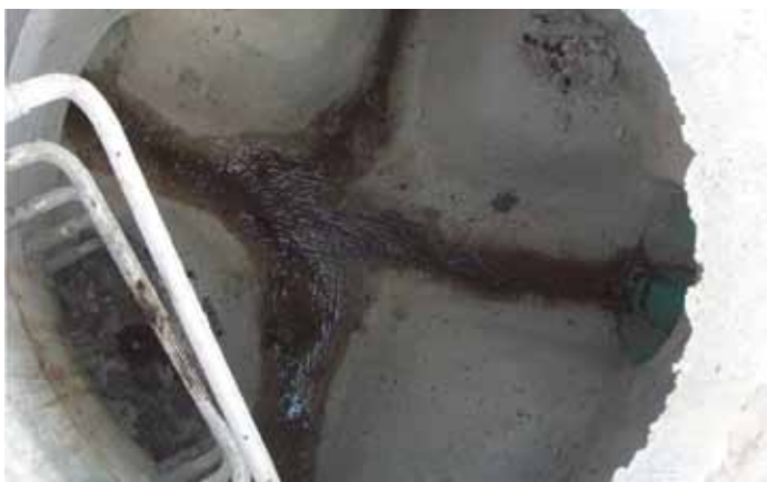
Figure 1 - Typical Field Benching
