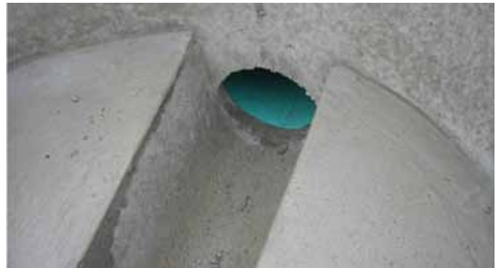
Figure 2 - High Quality Precast Benching
