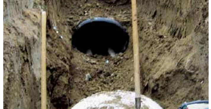
RCP being installed as HDPE is removed
