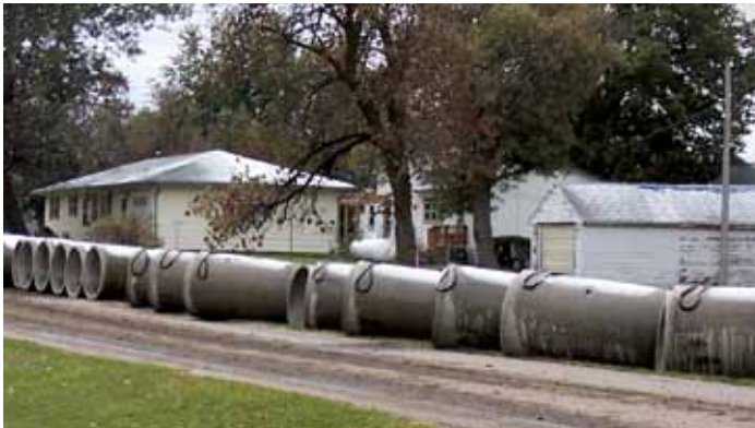
Reinforced Concrete Pipe with gaskets ready for installation
