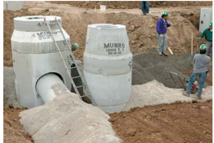
Reinforced concrete pipe, maintenance holes and catch basins for storm sewers, now underground
