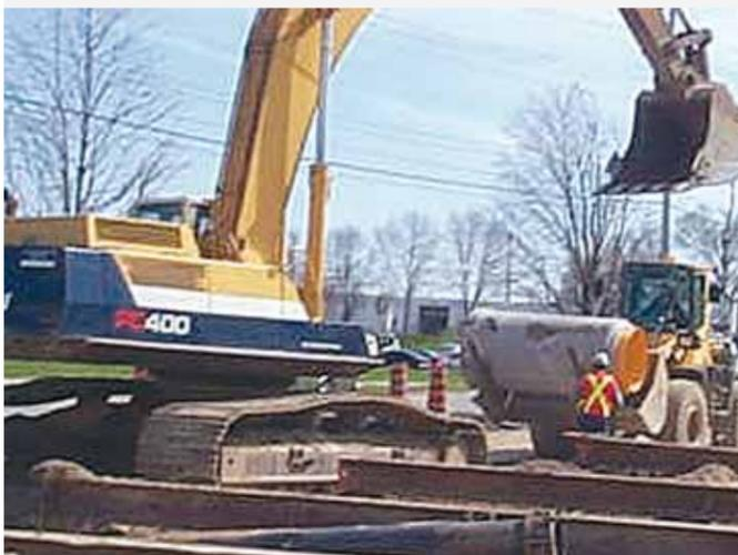
Concrete pipe installed through I-beams used to support existing buried services.
